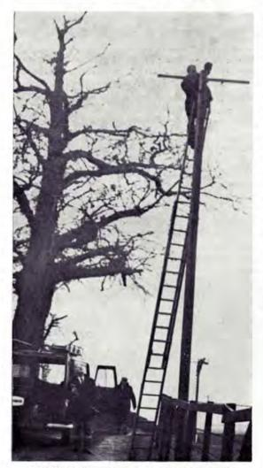
MANWEB linesmen at work on the spur line through Delamere Forest after trees crashed down on the conductors.
