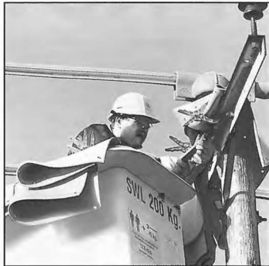
Hot Glove Linesman Hayden Bennett at work on Hawarden's town network.
