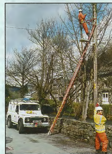
Preparations are made to secure a pole before it is removed.
