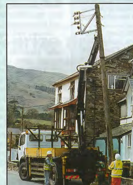
A mechanical grab is used in the last stages of removal.
