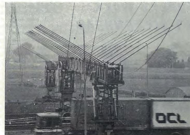
Overhead lines being drawn across the “Skycradles” as the motorway traffic rushes by underneath.
